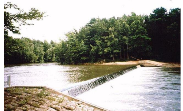
Low sill dam at Pools Bluff Sill
